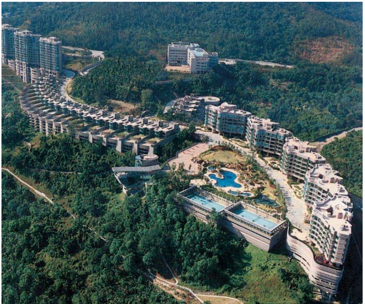
Deerhill Bay, Tai Po, New Territories, Hong Kong: Joint Investment Monitoring
